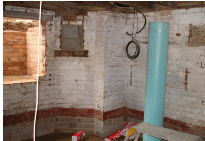
Minimal preparation is required to the substrate before cavity drain membranes are installed.
