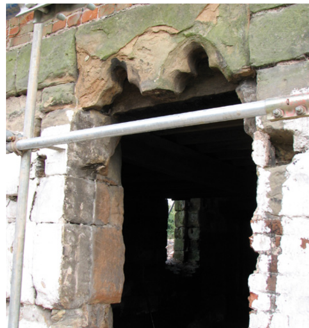
Original details have been retained in the development
