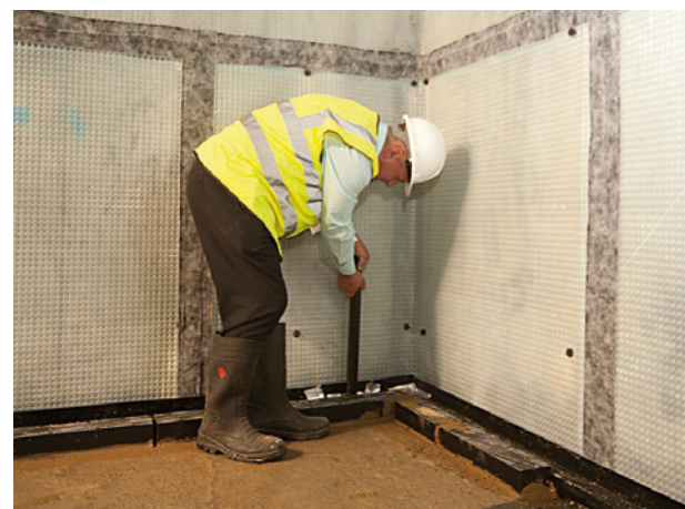
Installation of rodding eye extension to Aquachannel which will eventually protrude through block work for maintenance access purposes (close to sump pit which will house Aquapump Pro pump).
