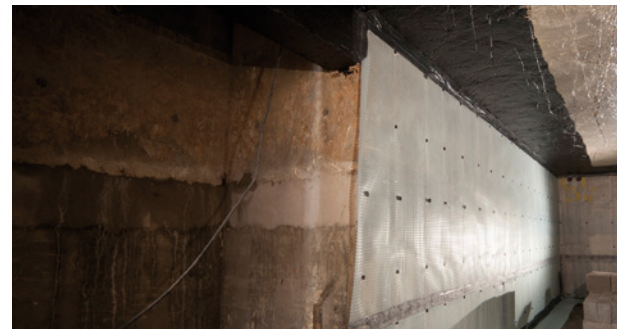
Triton TT Vapour Membrane was applied to the underside of the ground soffit and lapped 300mm down and behind the Platon cavity drain membrane to prevent and guide water migrating through the ground slab behind the wall membrane.
