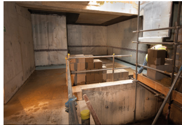
The complete below ground structure including the swimming pool was constructed using Triton's watertight concrete system.
