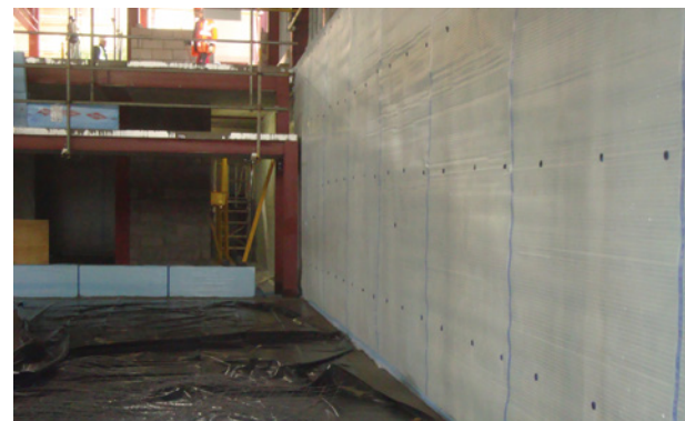
Platon Multi was installed to the walls
