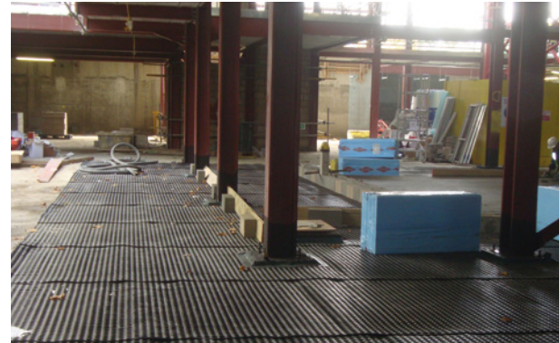
Platon P20 was loose laid to the new basement floor
