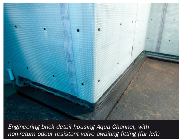
All perimeter walls were waterproofed with Platon Multi cavity drain membrane
